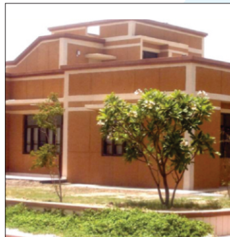
AMIT, Ph-II : Completion Year : March, 2007
