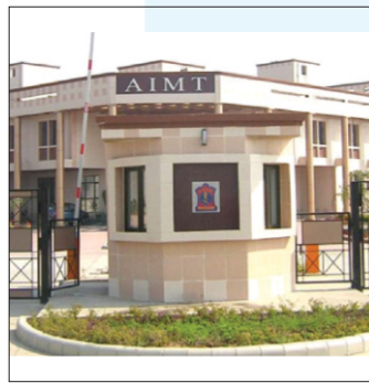
AIMT, Ph-I : Completion Year : March, 2005
