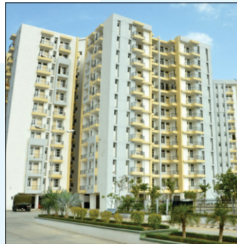
Jaipur, Ph-II : 572 DUs Completion Year : March, 2012
