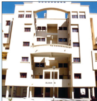
Hyderabad, Ph-I : 344 DUs Completion Year : July, 2001
