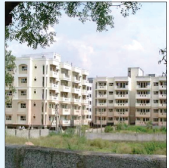
Hyderabad, Ph-II : 380 DUs Completion Year : October, 2012
